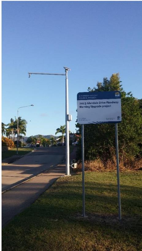
**Figure 3: Radar Roadway Flood Monitoring System installed at the Glendale Drive floodway in Townsville.**
