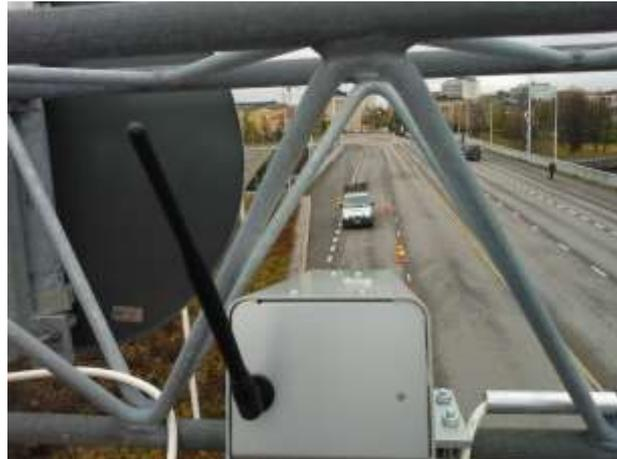
Figure 5. A laser radar affixed onto a gantry in the pilot site for measuring traffic and road data.
