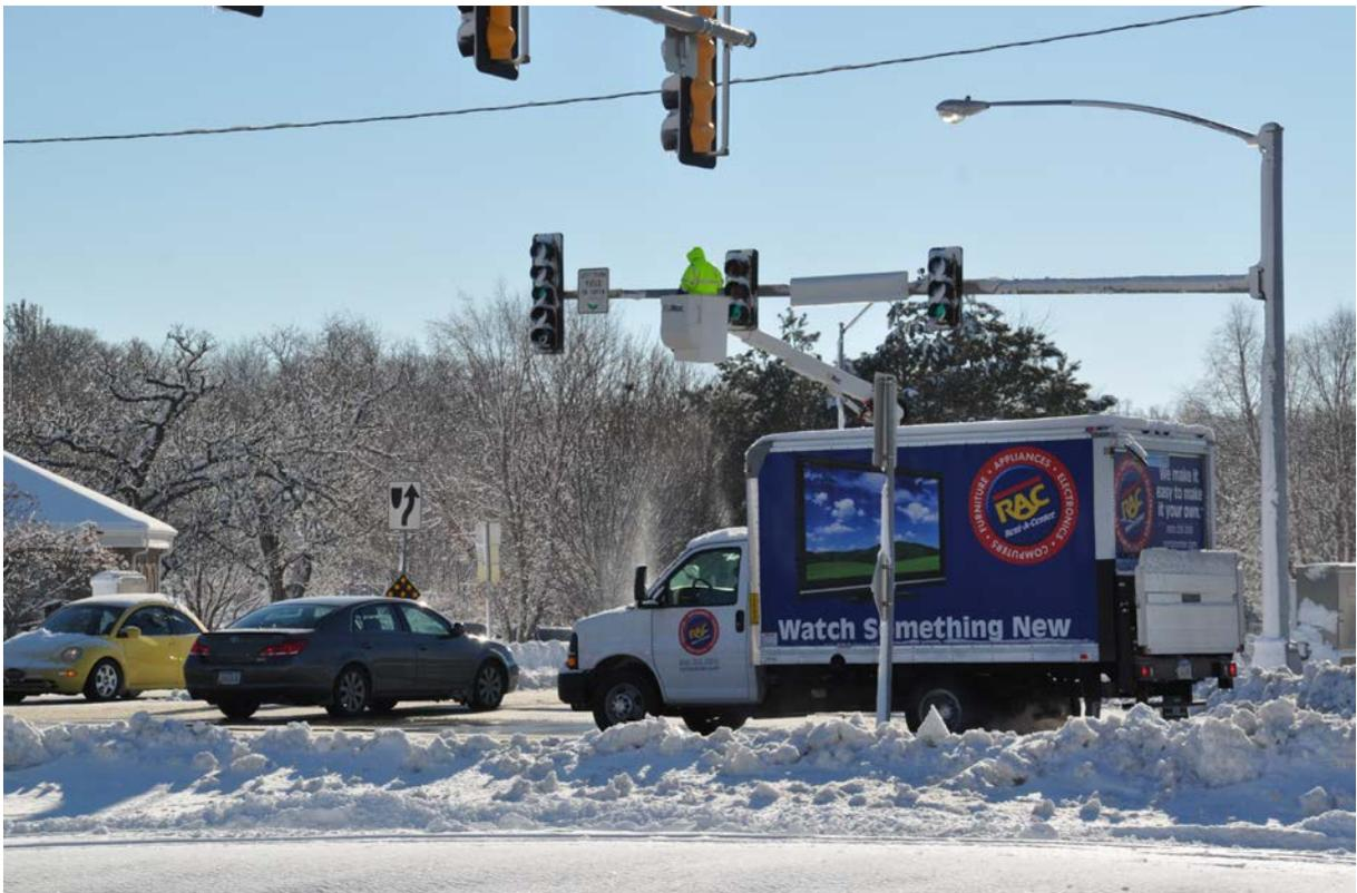
Figure 7: Snow Covered Traffic Lights Being Cleared of Snow
