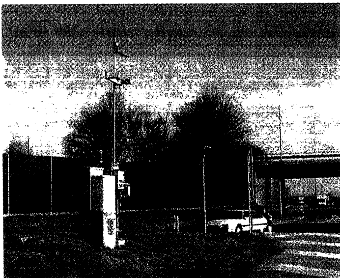
Installation of the instruments for the "Erlkönig" experiment at motorway A1
