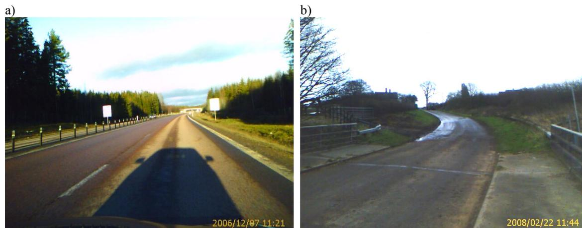
Fig.6. a) Differential drying on the E4 highway north of Gävle, Sweden (approximately 60.5°N); a) shows the effect of how heat fluxes from traffic dry the road surface on the heavily trafficked inside lane and b) Seepage across a minor road in the UK.
