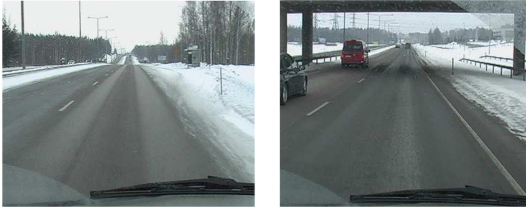
Fig. 4. The photographs are taken on the same time from roads near to each other and surface temperature at about  $-6^{\circ}\text{C}$ . There was light snow causing the wheel tracks on the left fairly slippery with friction less than 0.40, while on the right friction was over 0.60. The difference was caused by some more salt on the right. Interestingly, the area between wheel tracks remained practically dry on both roads despite the light snow fall.
