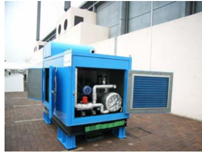
Bio Diesel Fuel(B100) Power Generator
