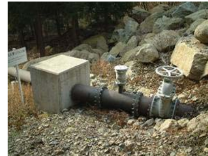
Small size Hydropower Generation using Tunnel spring water
