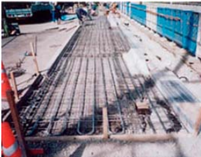
Execution case of the subterranean water heat returning style non-water sprinkling melting snow institution
