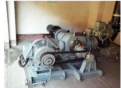
Small size Hydropower Generation using Tunnel spring water
