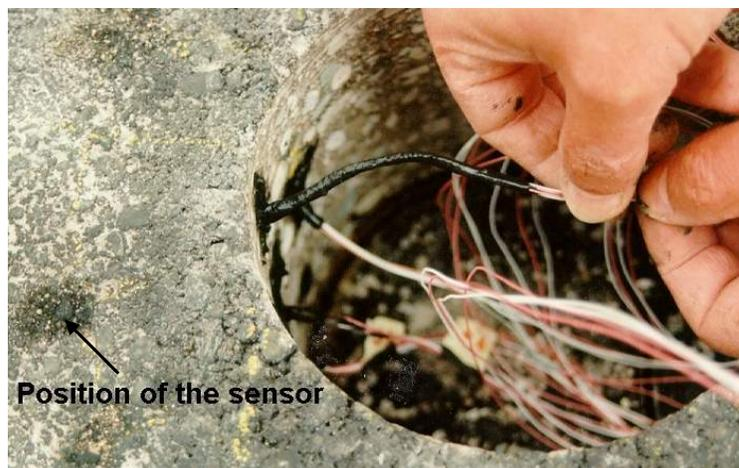
Figure 2: Installation of a sensor for roadway surface temperature on the roadway surface
